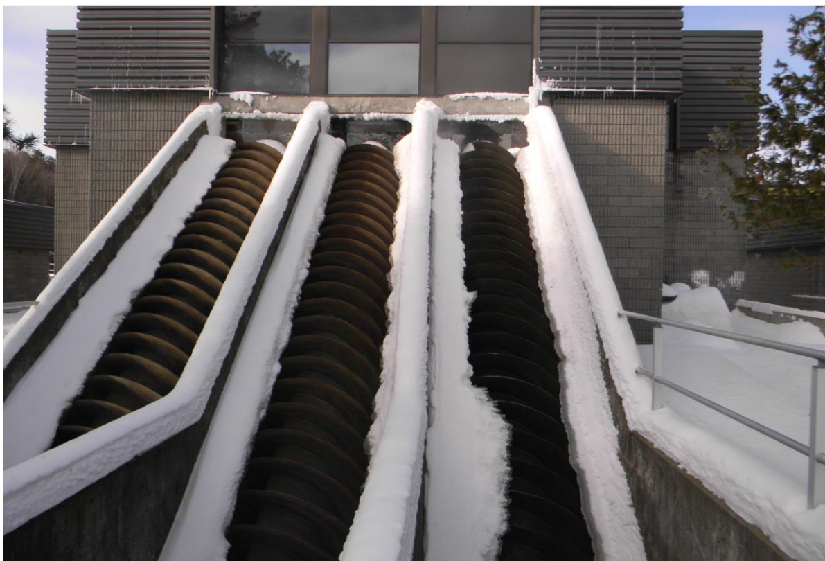
Figure 3 - Wastewater Treatment Plant (Screw Pumps)
